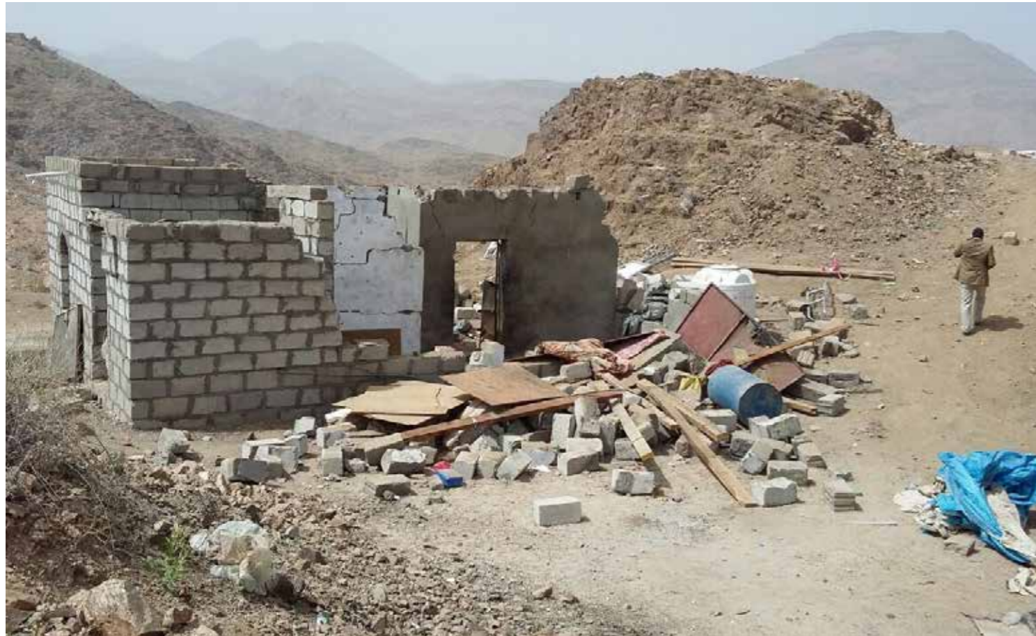
Photo - House destroyed by a missile
